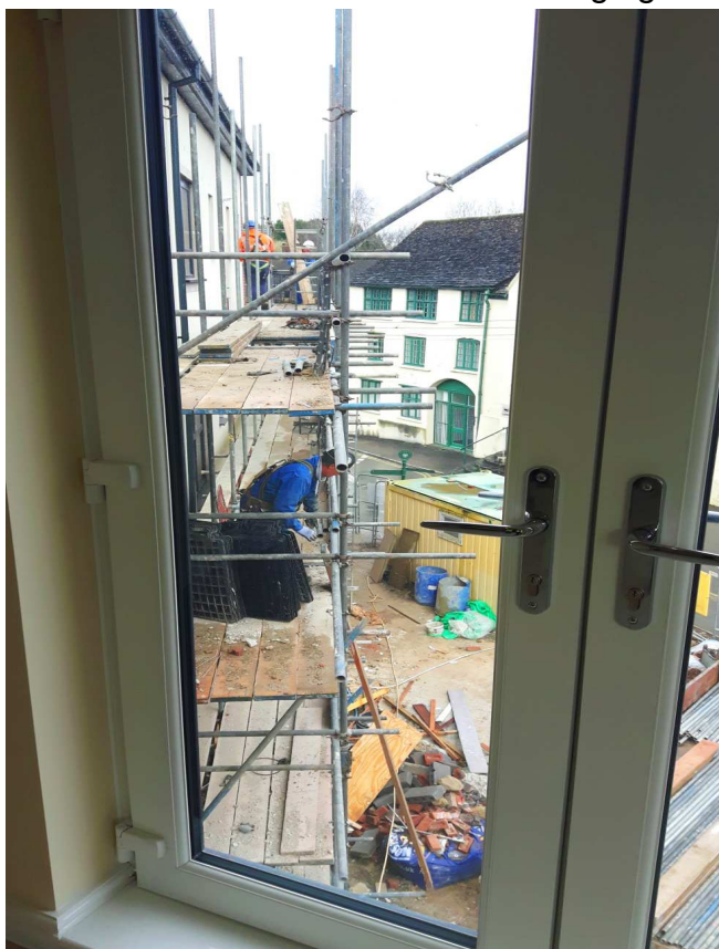
Affordable flats under construction in Dursley, 2017
